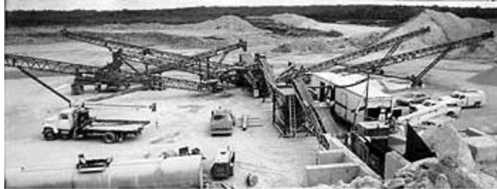
The Olathe Aggregate operation includes a Pioneer ® 4654 HSI, a Pioneer 5260 HSI and a Pioneer 6' x 20' three-deck screening plant.
